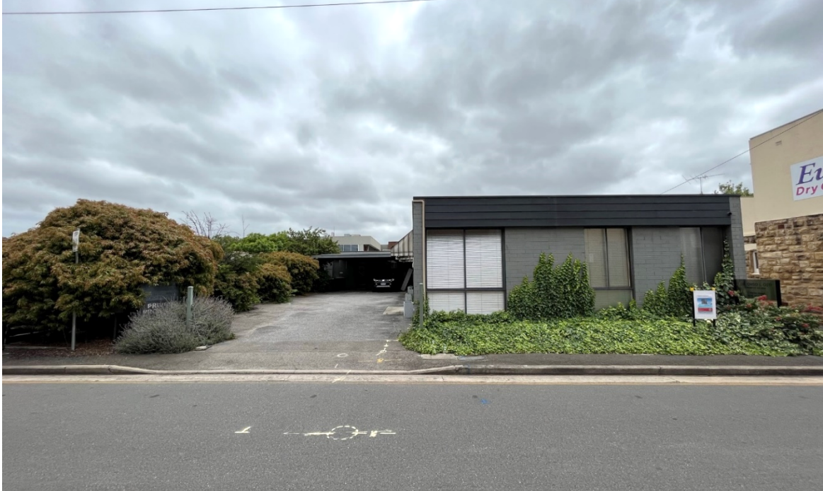
Photo 3.1 – subject site viewed from Walter Street looking north
